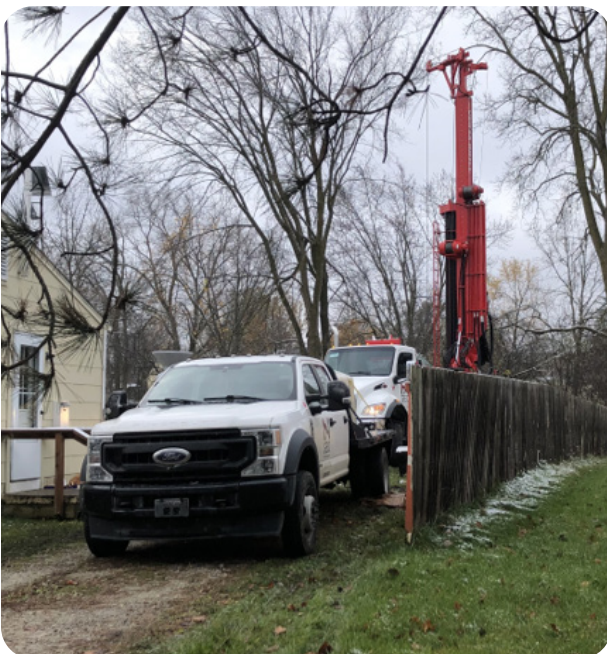
Geothermal rig at the Bryant Community Center drilling the vertical wells for the Center's geothermal heating and cooling system.
